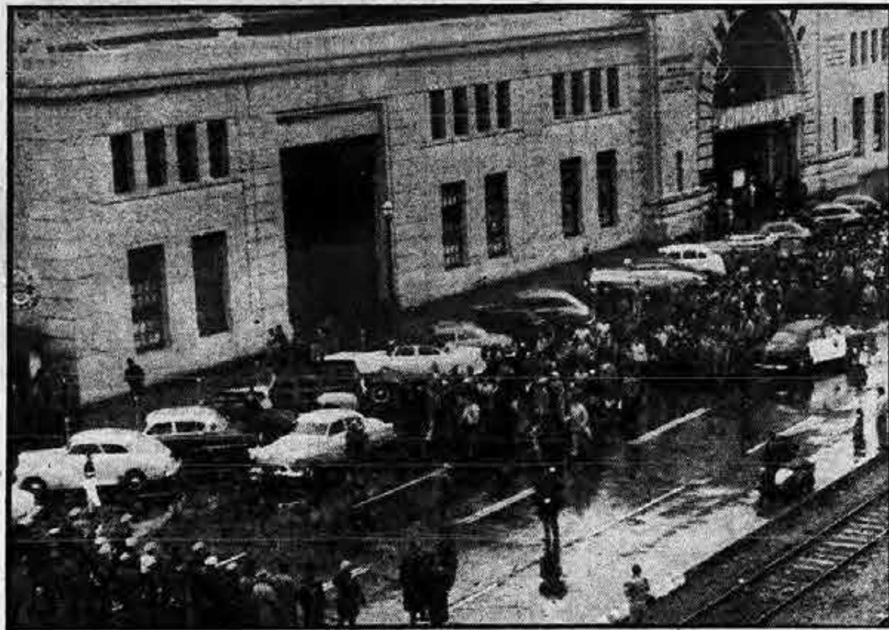
A line of police, with billyes and clubs ready, stands waiting as a long line of SUP, MFOV and MCS-AFL demonstrators march down the street toward Pier 39 in San Francisco. Demonstrators were headed toward Bryson-Bridges squads at the pier who had roughed up Aleutian crewmembers. Cops used their clubs to stop demonstrators and to protect Bryson-Bridges squads.
