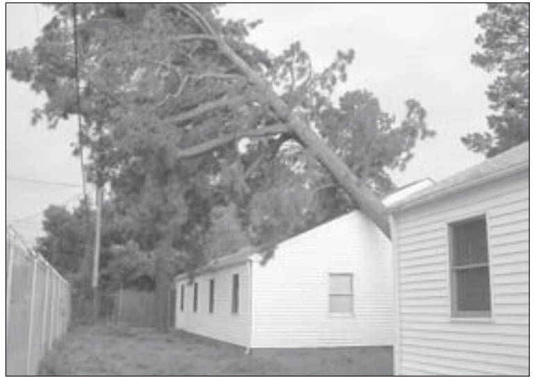
A number of trees at the Paul Hall Center fell during the storm, including this one which landed on a classroom building.
