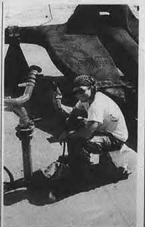
OS Kevin Young chips a fire monitor on the vessel's bow.
