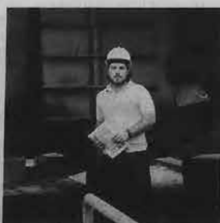
Tankerman Scott Hardin performs some needed repairs to the tug Achilles , drydocked in Lake Charles.
