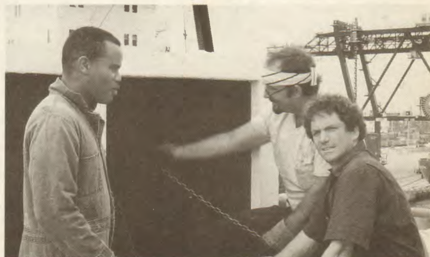
Installing repaired cargo fans aboard the roll-on/roll-off vessel are, from left, DEU Levi Rollins, QMED George Habinger and QMED J.R. Cirafisi.
