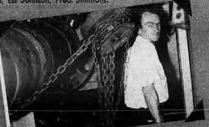
Ship's delegate Jim Cochran watches the raising of the main propulsion shaft while the Cuba Victory was undergoing repair work.
