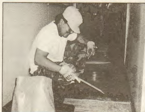
Replacing tile inside the vessel is AB Nestor Agcailli.
