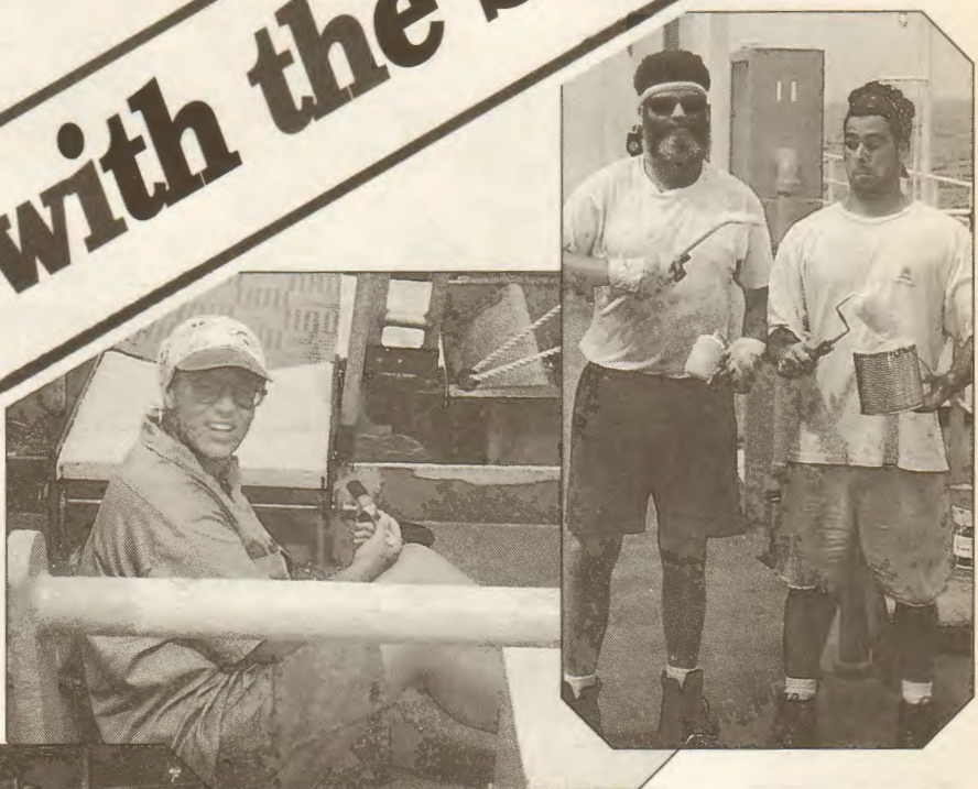
The OMI Columbia gets a fresh coat of paint by members of the deck department. Above left is AB Kathy Chester; above right are ABs Stephen Votta (left) and Randy Senatore.
