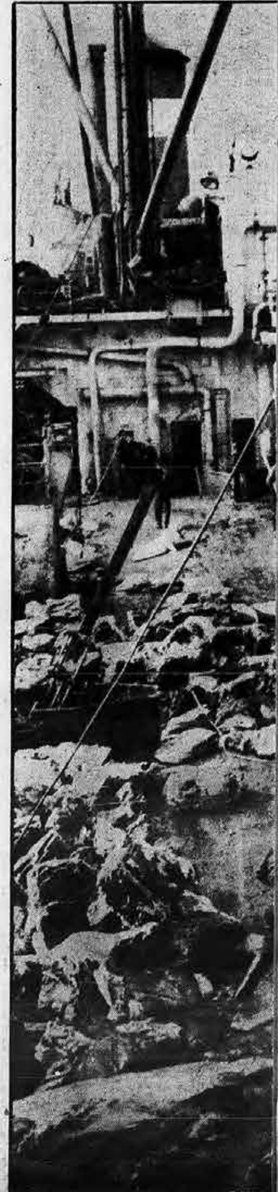
The hval kla, or "grab" reaches skidway to seize a whale's tail for the animal inboard.
