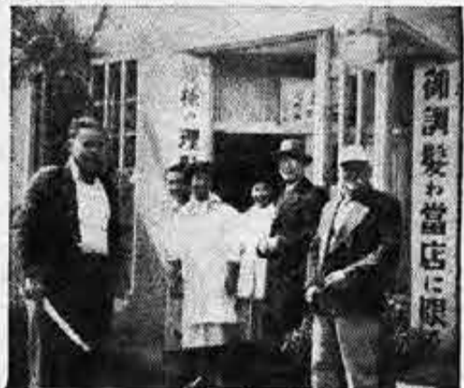
Entrance to barbershop serves as meeting place for Seafarers and Yokohama citizens.
