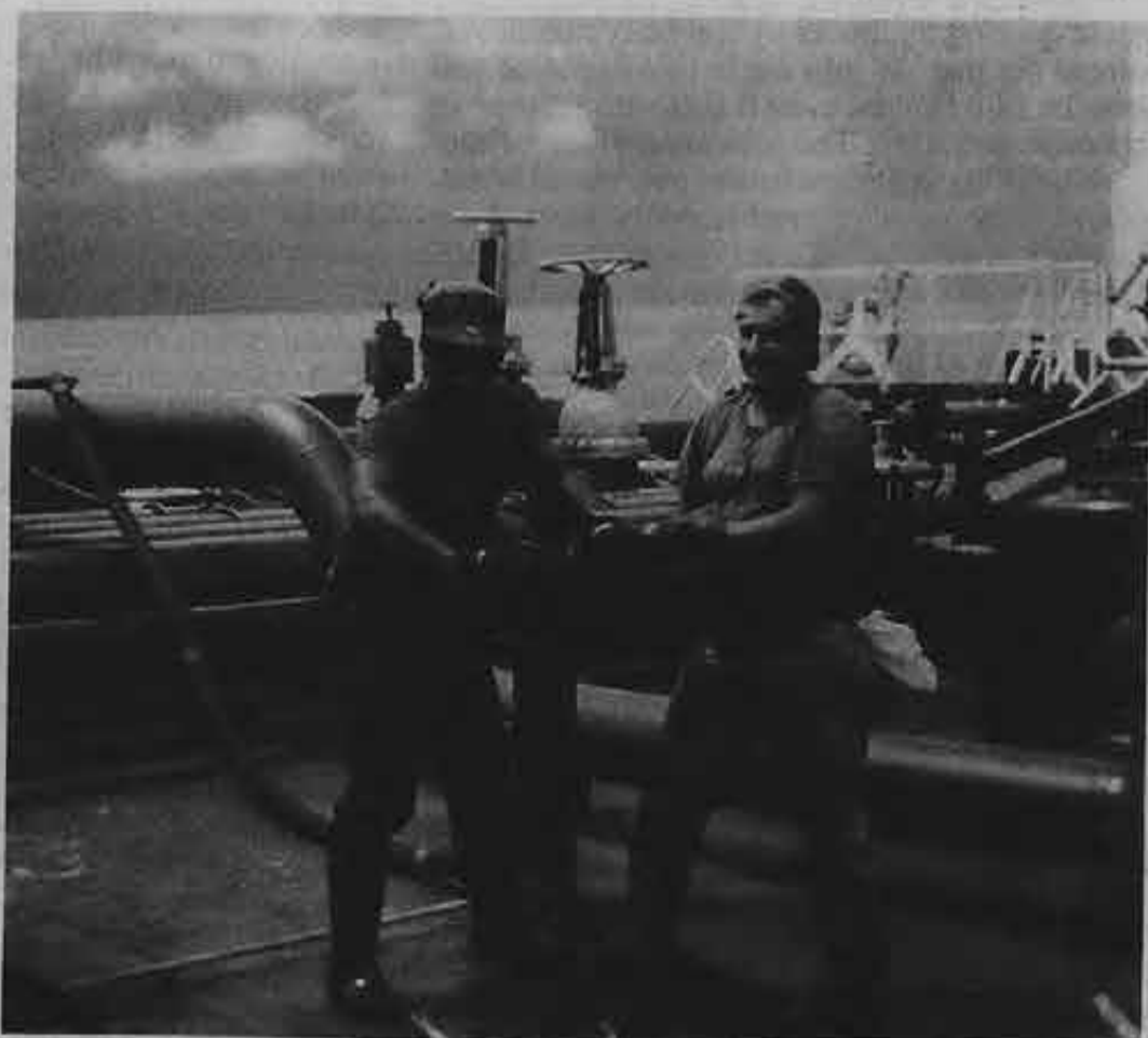
Tightening the butterworth plate before arrival in port are, from left, AB Terry Cowans and AB W. Lopez.
