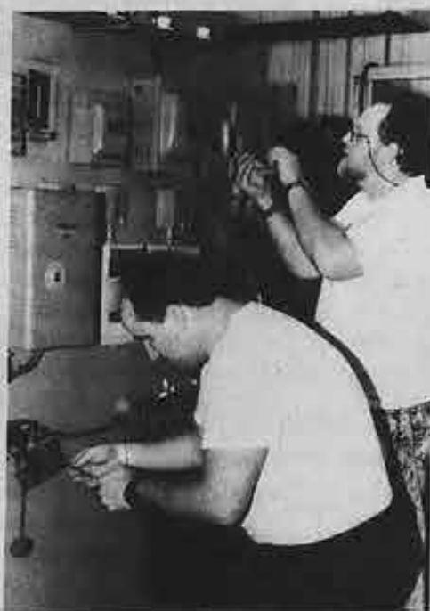
Engine department upgraders Robert Hamil (left) and Charles Betz wire marine receptacles and lights.
