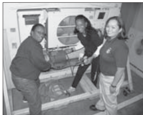
Engine Room Seafarers Emma Porter and Annie Walker and Phase III Unlicensed Apprentice Paula Gomez test a part during an engine utility class.
