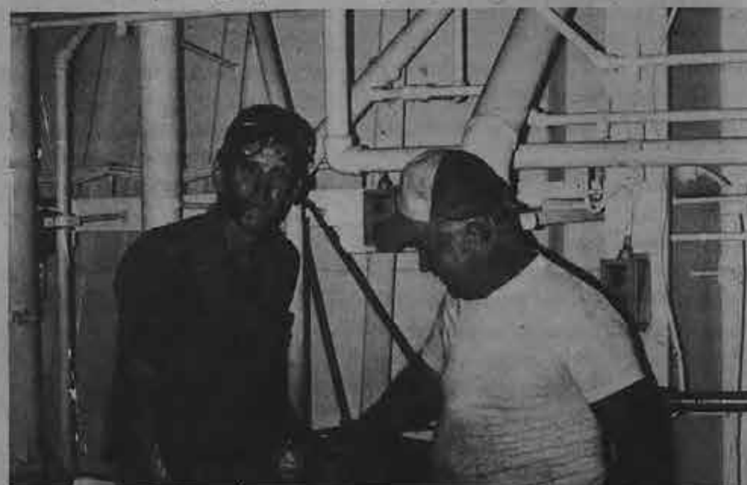
QMED Jimmy Slay and QMED/Pumpman Dave Norris discuss the advanced technology found in the engine room of the ITB Moku Pahu .
