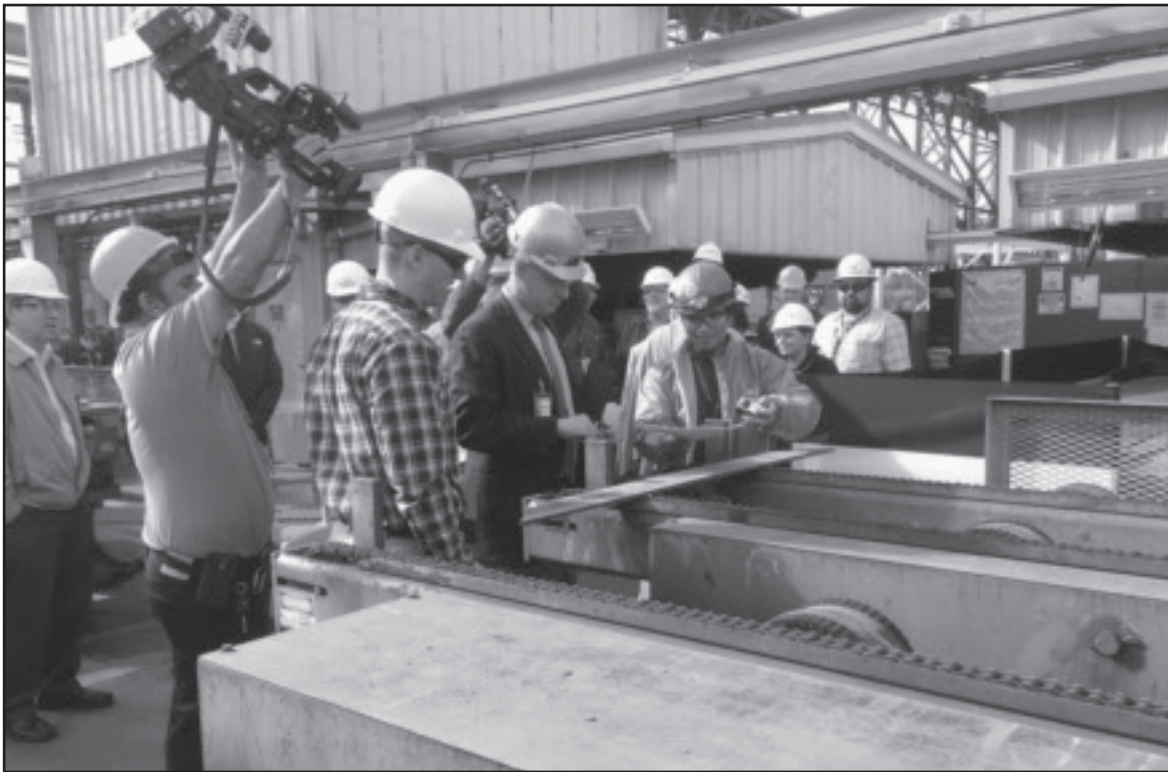
A ceremonial steel-cutting marks the start of construction of another Jones Act tanker at NASSCO. (Photo courtesy General Dynamics NASSCO)
