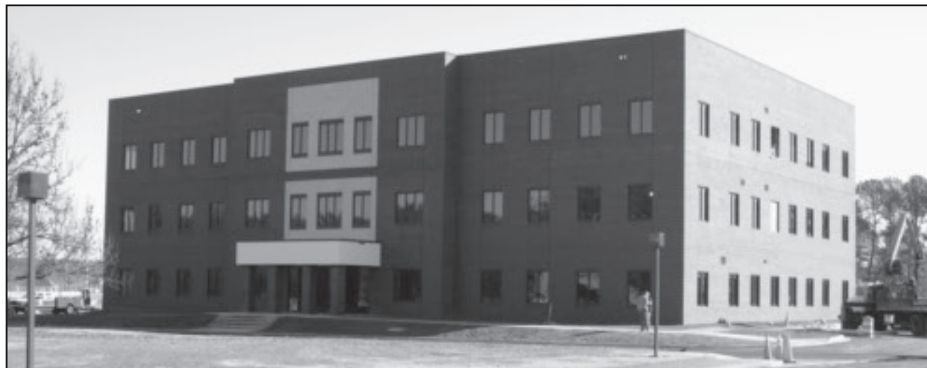
The new Claims Building is nearing completion.
