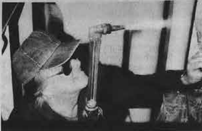
QMED John Kelley repairs a leaking pipe near the crew's quarters.
