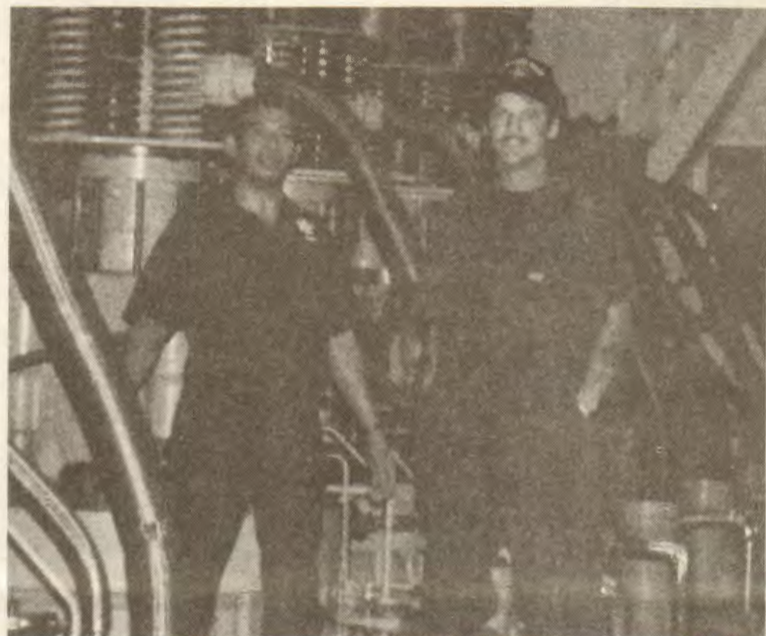
Conferring next to a diesel engine aboard the Shughart are QMED Robert Dupaya (left) and Bosun Robert Walker.
