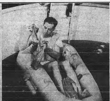
man squeezes the upper portion of the bag, containing sea water and a filter sack. This disperses chemical in the water and removes the salt. In the center picture the saltless water is transfered into the second bag for the purpose of removing the sedium. After the second bag has been
