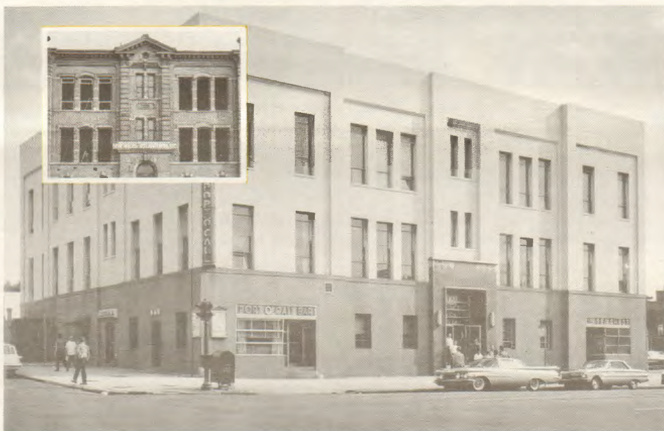
Job opportunities for SIU members expanded so rapidly that the union was forced to move to a new headquarters building in Brooklyn. "Frenchy" Michelet oversaw the repairs (inset).
