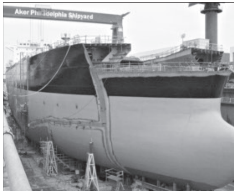
The hull of the second tanker in the series (above) is nearing completion with only two sections remaining. As of early February, the deckhouse had been mounted atop the ship and was undergoing outfitting, while the piping systems in the engine room and main deck were being completed.
