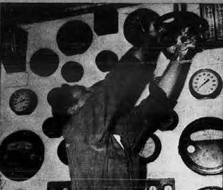
Seafarer Wayne Kidd of the Engine Department is busy opening the root valve with the Hagen board showing in the background.
