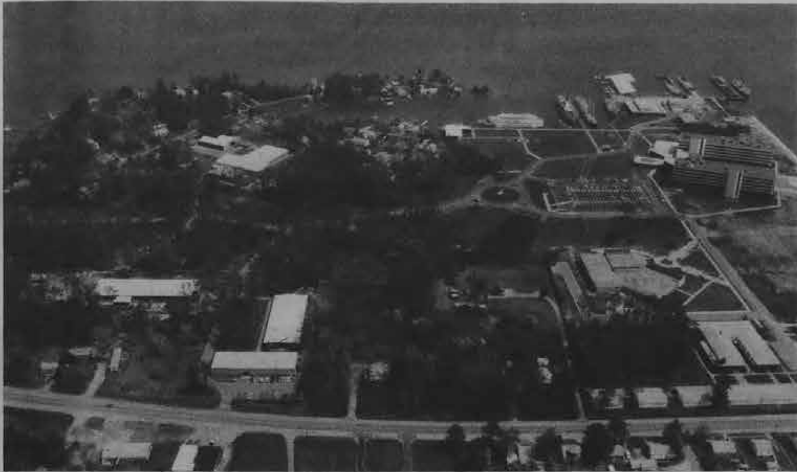
AERIAL VIEW of the Seafarers Harry Lundeberg School of Seamanship.
