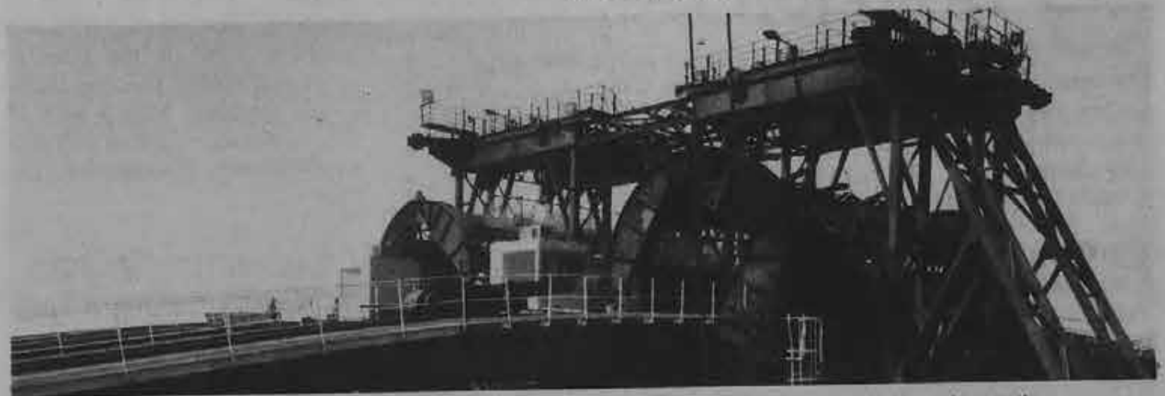
The Harriette regularly loads on coal cargoes brought by rail to this adjacent train trestle.
