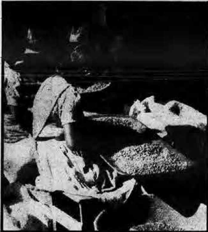
More drying follows the hulling operation, after which the "green" or unroasted coffee is graded for size. Although machines grade it automatically, it is re-sorted by hand (above) so that only the finished coffee beans remain for bagging and export.
