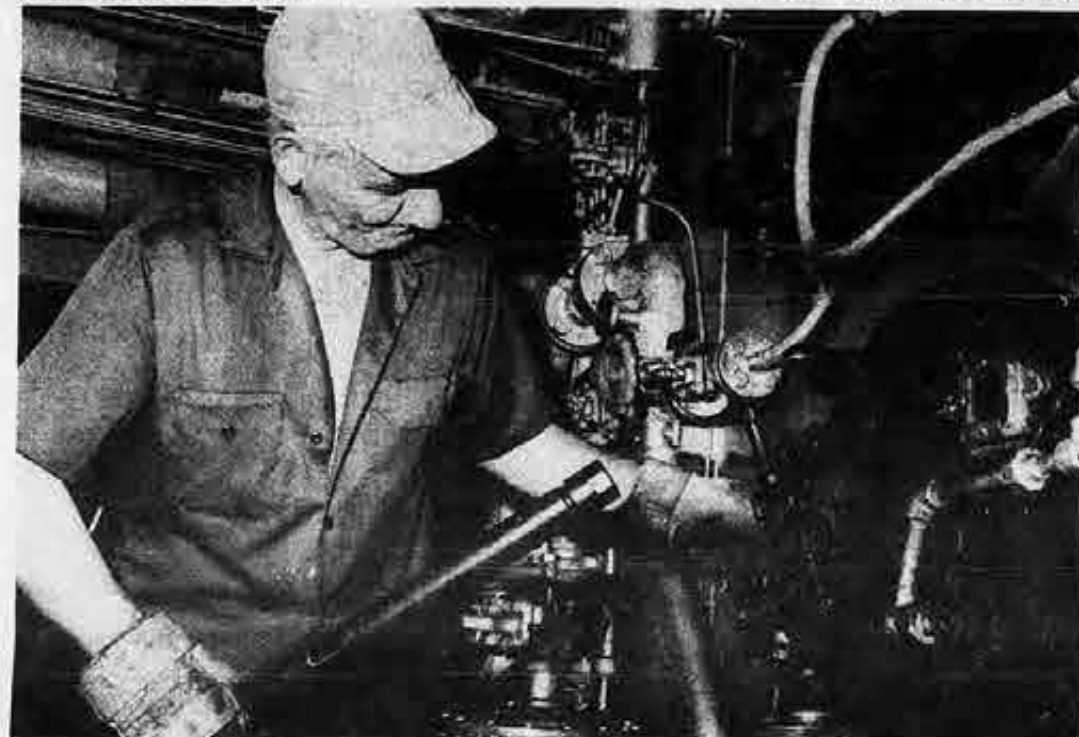
Fireman Donstancino Ruggiero changes the burner rod in the engine room on the largest cable ship in the world.
