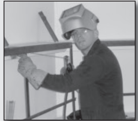
Pumpman Tom Bain is busy welding in the steering gear room.
