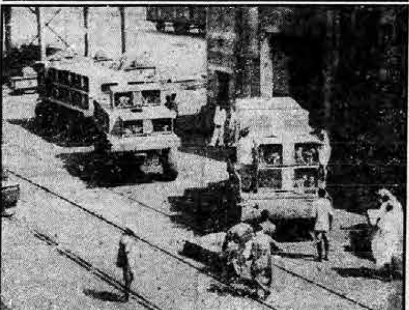
Charlie, above, in one of his rare moments of inactivity, sits quietly aboard the Steel Navigator near one of its fire stations. Below, some of the 600 monkeys which were loaded aboard the ship roll along in their cages under the watchful eyes of native keepers in Calcutta,
