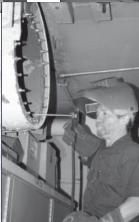
Right: QMED Ken Pell prepares to weld in the engine room.
