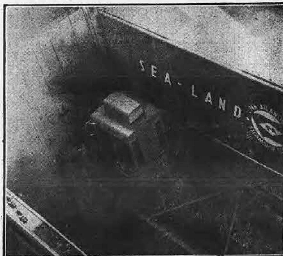
After depositing and releasing trailer body, the traveling lift emerges from the hold for another 22-ton load.
