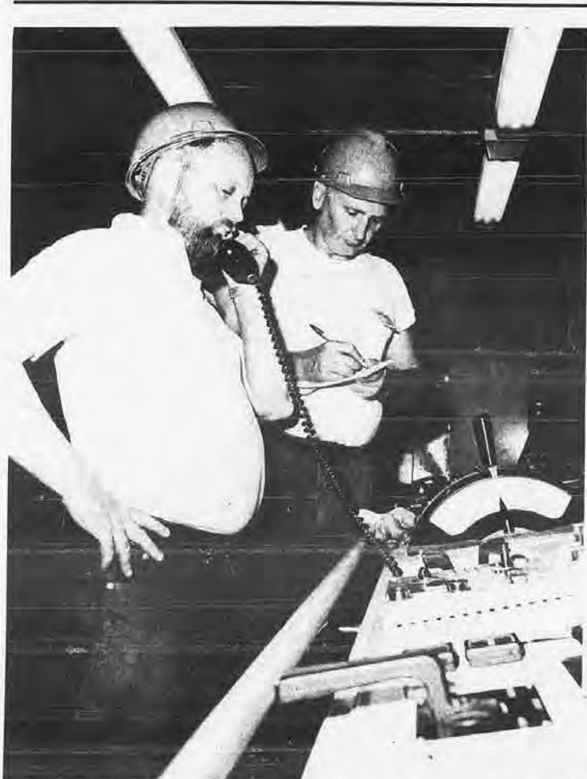
QMED's Tom Curtis, left, and Wilburt Hyder will be seeing plenty of the LNG Gemini's automated engine room.
