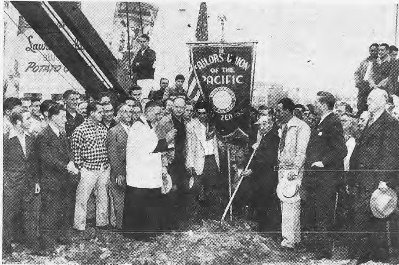
From humble beginnings on the Folsom Street Wharf, the Sailors Union of the Pacific has grown to magnificent proportions. Now the organization is engaged in a building program, the first evidence of which is the Headquarters Building, being erected in San Francisco. Pictured above is the ceremony to celebrate the breaking of ground on the site at the foot of Rincon Hill. As Rev. Edward B. Lenane blesses the site, Nick Jortall, oldest living SUP member, turns the first spadeful of earth. Harry Lundeberg, Secretary of the SUP and President of the SIU, is standing next to Rev. Lenane.
