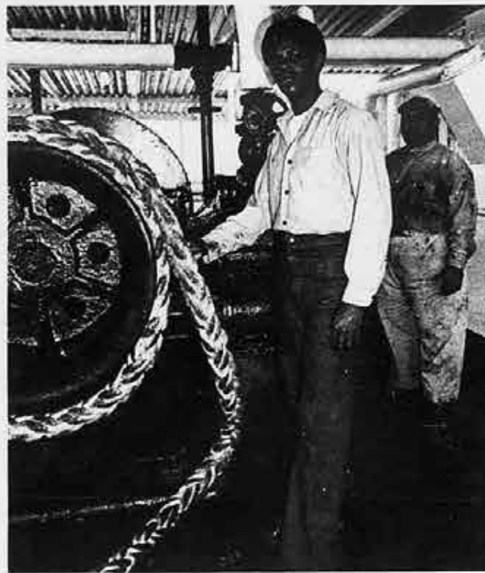
Ordinary seaman M. Sherard (foreground) uses a winch to wind in heavy-duty lines topside, with an assist from C. Figueroa who sails as deck maintenance man.
