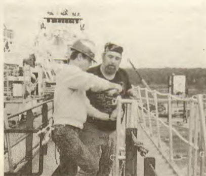
Watchman Jim Smith (left) and Bosun Terry Henretta put finishing touches on the new gangway.
