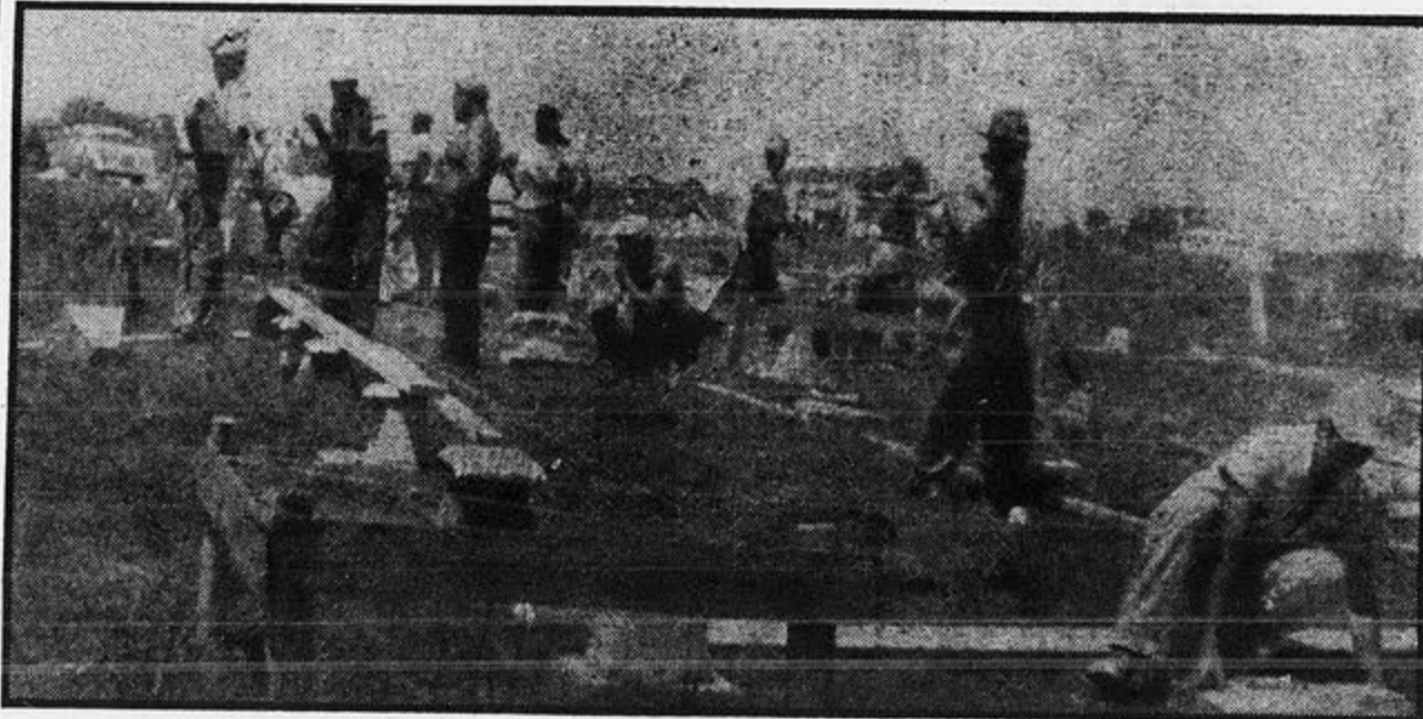
Foundation for new home in Cameron goes up as soon as gang arrived. Even bus driver W. A. Polk pitched in, shedding his uniform to lend a hand. Homes were put up in other flood-stricken towns with some of the volunteers working far into the night under floodlights to make the target of completing a number of houses each weekend.
