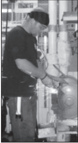
UA Chad Bruch grinds a pad-eye for welding.
