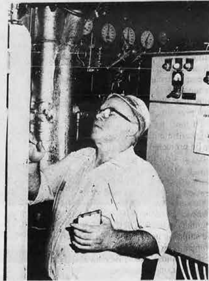
Taking routine readings in the ship's engine room is Seafarer Clifford Sewell, sailing oiler maintenance. The Delta Argentina is carrying heavy farm equipment to ports in West Africa.
