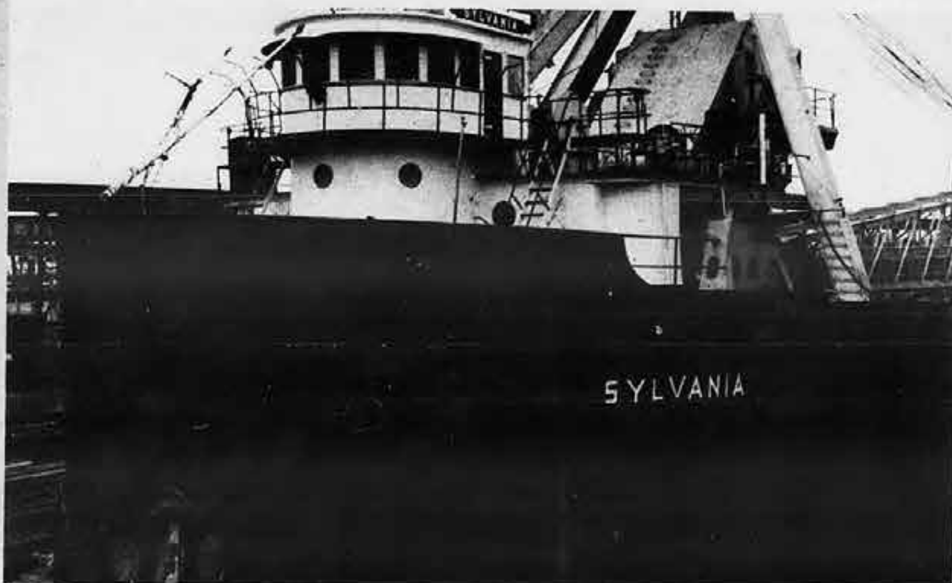
The Sylvania (Tomlinson Steamship Company) is high and dry in a Toledo drydock for survey of her hull during her annual inspection. Typical of the Great Lakes fleet, the Sylvania is more than 40 years old. Also typical, this self-unloader is fueled by stoker-fed coal.
