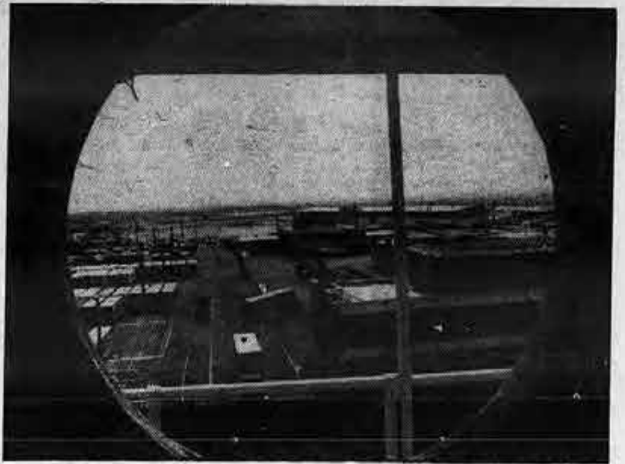
Porthole view from one of the Sea-Land's containerships shows the heart of the SIU company's new $22 million headquarters and terminal in Port Elizabeth, NJ. The company's yards can handle 2,000 trailers at one time.
