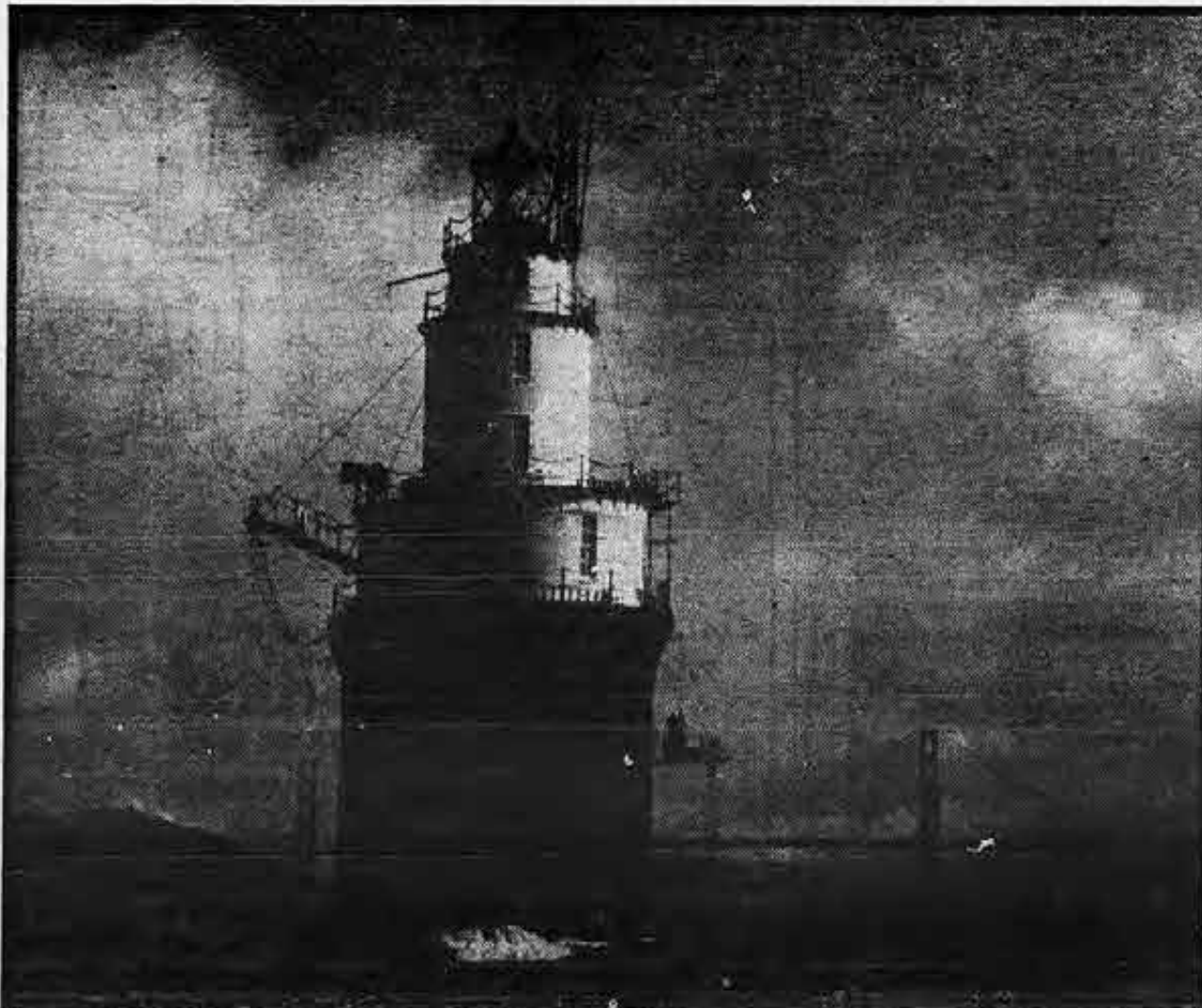
The Mile Rocks Lighthouse stands one-half mile off Landsend, in the Golden Gate, and within view of San Francisco. It was completed in 1906, after considerable difficulty caused by the heavy seas and strong currents occurring at this point. The rock upon which the lighthouse stands measures only 40 by 36 feet at high water.
