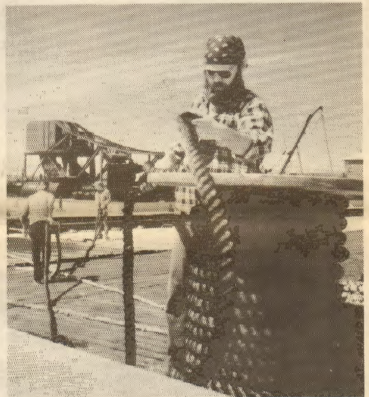
Engineer John Tanner (foreground) and the rest of the Peggy S crew load new line aboard the tug.
