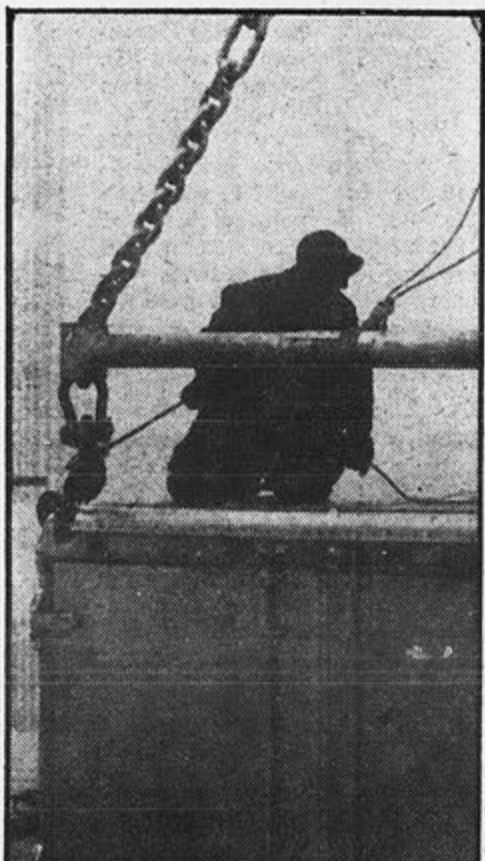
4. Longshoreman removes hook from rings on top of trailer. Remote gadget can also do job.
