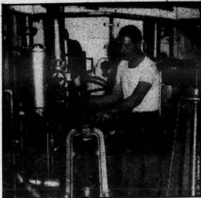
William Bowles, oiler, opens sea suction valve so water can cool condenser.
