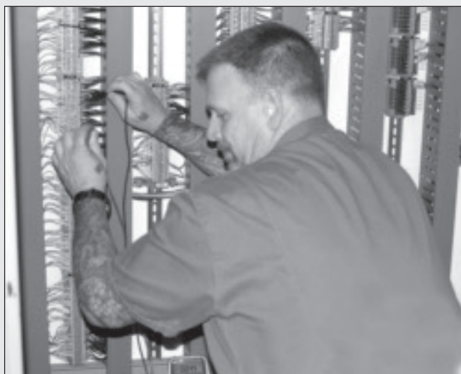
Electrician John Hunt does some troubleshooting.
