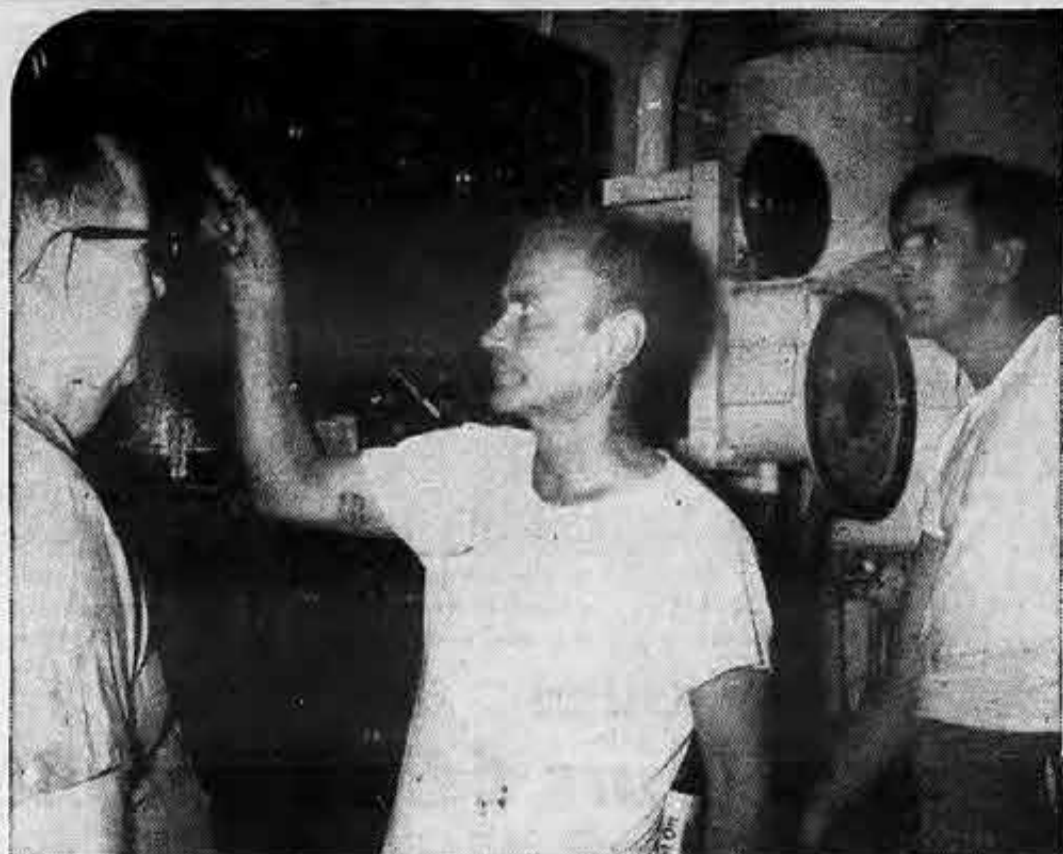
Keeping a watchful eye on the engineroom gauges (l-r) are J. S. Skidmore, 3rd engineer; Paul Cavan, oiler, and J. Gilbert. After loading in Baltimore, the Topa Topa (Waterman) headed for Greece.
