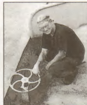
Pumpman Dave Bouda checks a valve.
