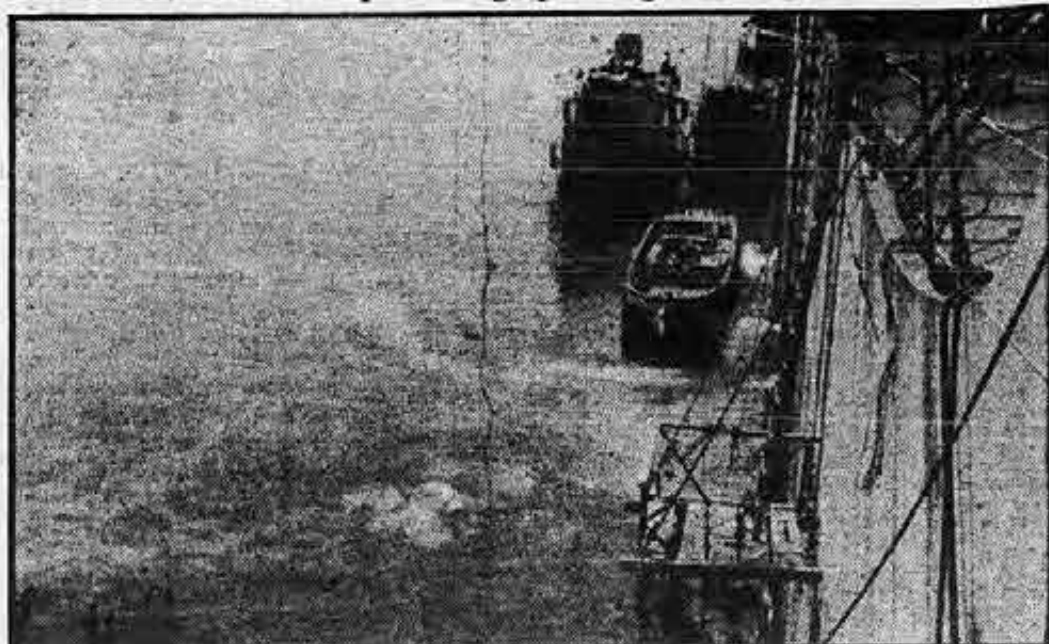
Navy small craft alongside San Mateo were used by salvage experts and divers who placed explosives for blasting rock from under the ship. Six special salvage ships were used for the work.
