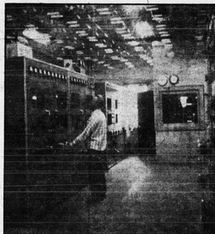
Engineer at Hicksville, LI, transmission station shows radius of voice broadcast on world map (far left). As broadcast begins, he plugs in board (center), and controls voice volume. Control panel (right) shows all gear working properly. Facilities here can handle 60 different transmissions at same time.
