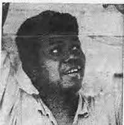
David Maffia, electrician, took care of the wiring.
