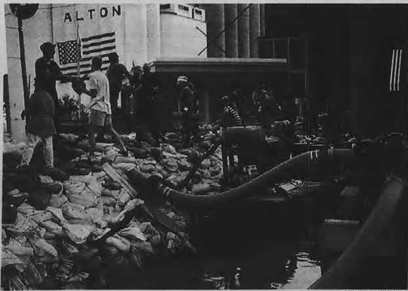
Alton residents and Illinois National Guard members add more sandbags to a wall created to keep floodwaters out of the city's business district. This scene is two blocks from the SIU-crewed Alton Belle . AP by Michael Winokur
