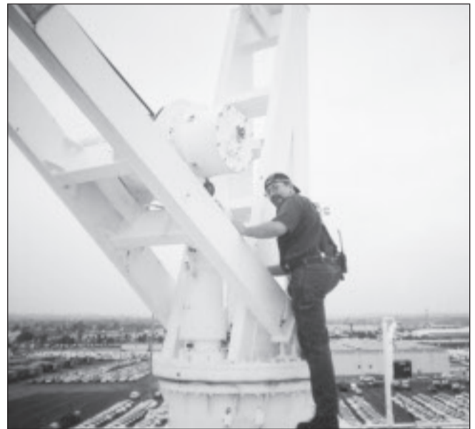
Repairing the crane aboard the Jean Anne is Electrician David Cutro.
