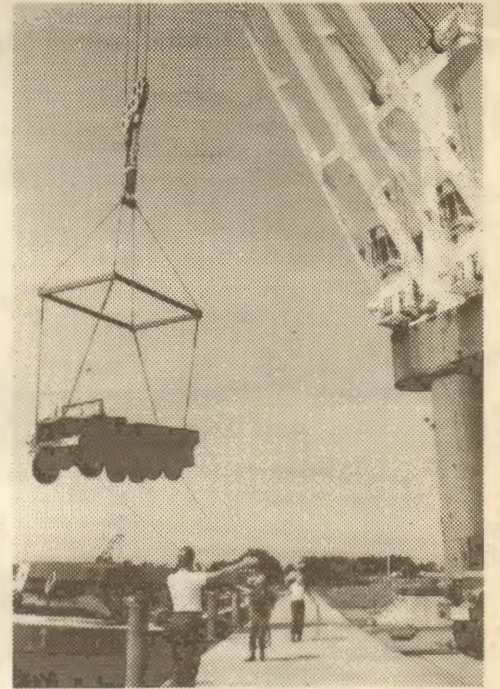
A military truck is lifted clear of the barge as the signalman gives the slew signal which will move the crane to the right.
