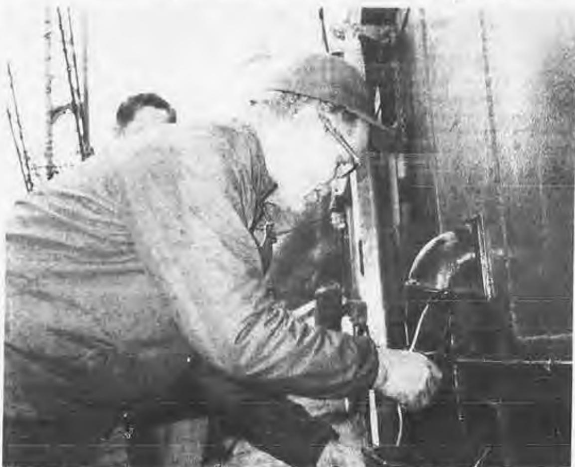
SIU Oiler "Dean" Sams, a 22 year book man, repairs an electrical deck fitting on tug America (Great Lakes Towing) in Detroit.
